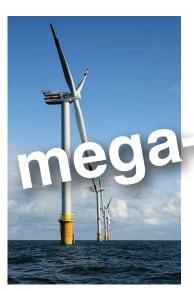
This offshore wind turbine near Belgium has a power capacity of nearly five megawatts!
